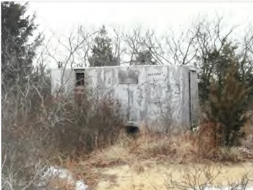
Figure 3.12. View looking north at a post World War II trailer, Batteries Engle and Peck. Northeast of Battery Engle, a communications trailer sits abandoned. The trailer is a frequent target for graffiti (Olmsted Center, January 2009).
